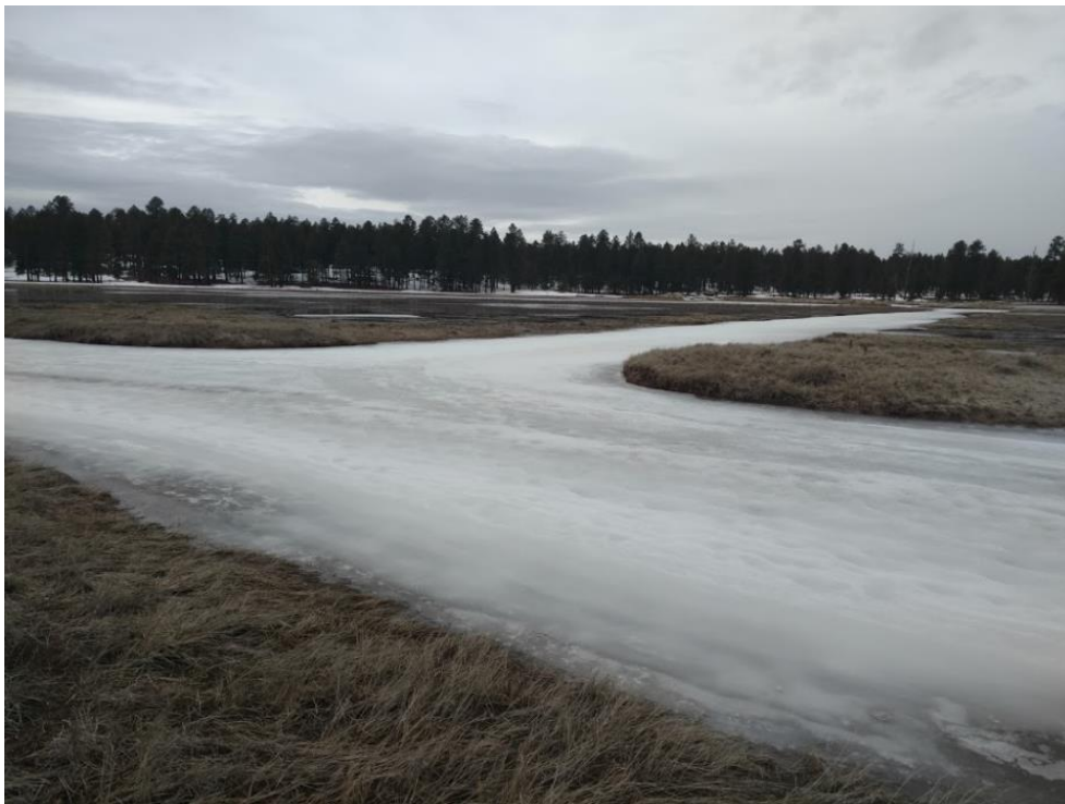
Appendix Figure C6: Trenches in the unrestored area covered by ice during the winter. (February 17 th , 2017)
